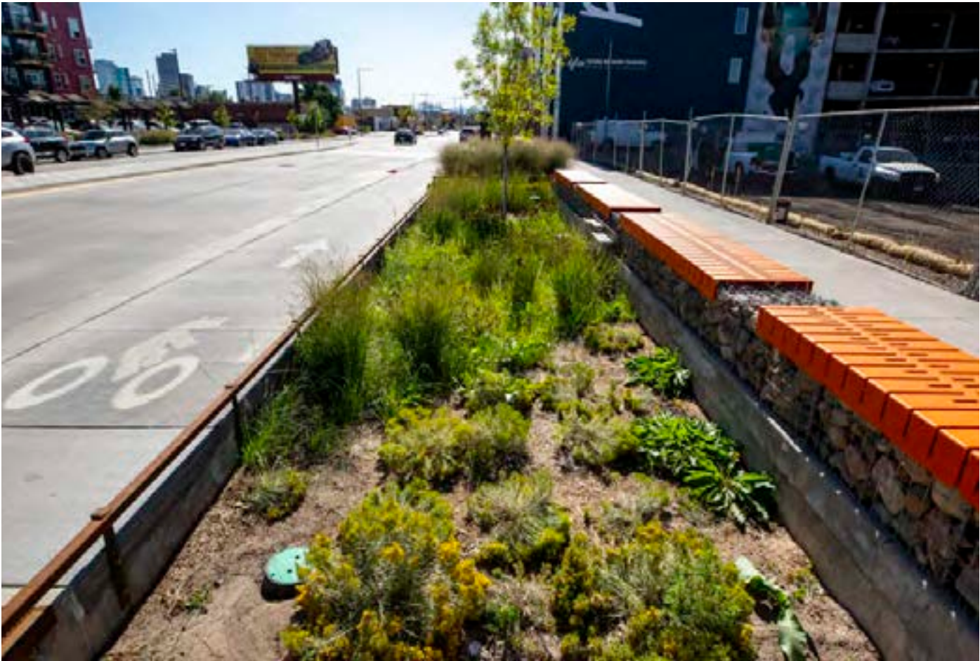
Green infrastructure in Denver can help cool streets while filtering pollutants and reducing runoff during storm events.
