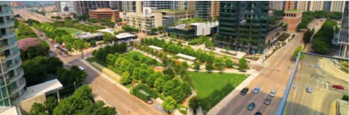
Figure 7.7: Example of an Arterial Lid
